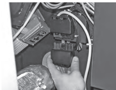
Fig. 160 Disconnecting the blower plug
