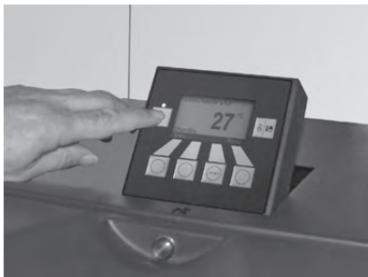
Fig. 154 Switching off FireWIN
