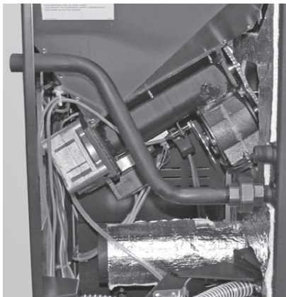
Fig. 22 Sealing the screw connection and fitting the flow pipe
